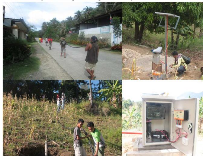
Figure 3. Transporting the assembled sensor column from the location where it is assembled to the deployment site (top left) and installation in the borehole (bottom left). The solar panel used to power up the system (top right) and the enclosure box that contains the battery and other electronics (bottom right).
