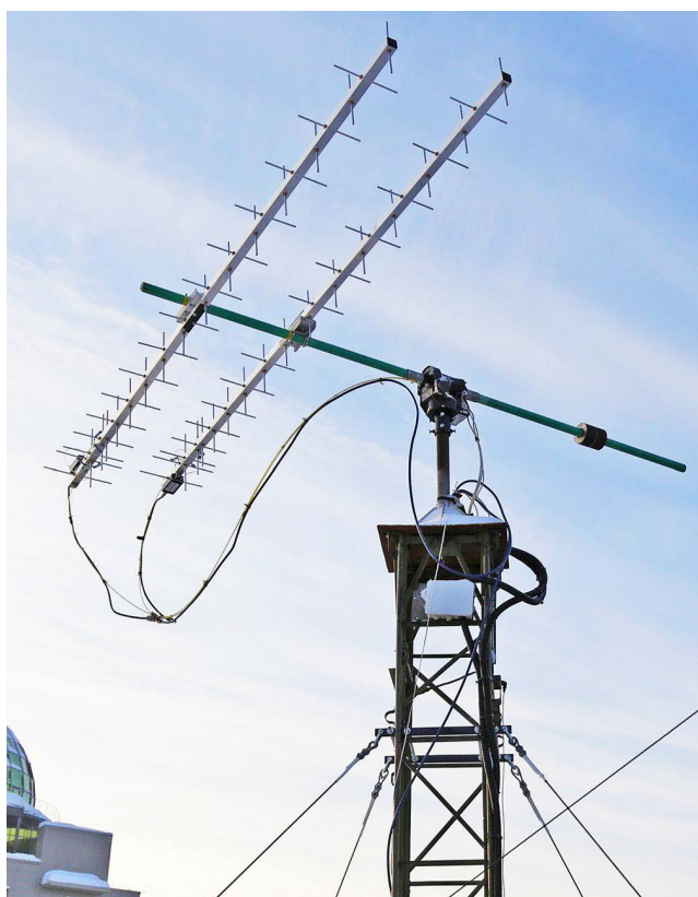
FIGURE 3. Ground station antenna.
