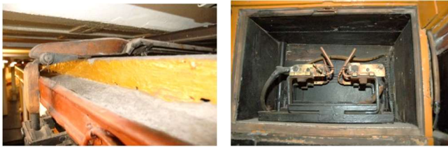
Fig. 15.: Sliding contact and wooden insulators and spark-gap at the entry to the carriage-body (URM)
