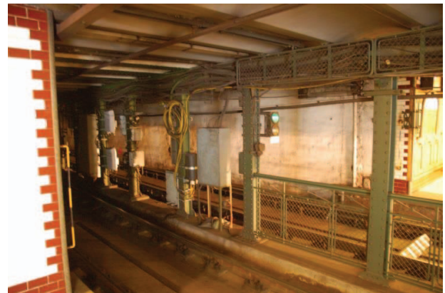
Fig. 7.: Tunnel start at Vörösmarty street station
