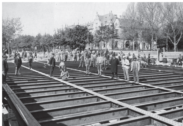
Fig. 5.: Construction of the station “Arena street” (fortepan.hu)
