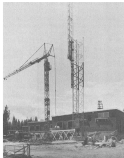
Figure F-3. The Tampere mast under construction.
