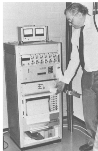
Figure F-5. Vibration of the masts and guys are continuously monitored by automatic logging equipment.
