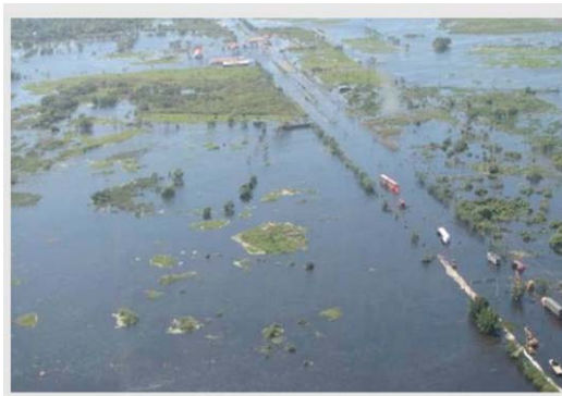
Fig.1: Federal road 180D totally submerged. Transit problems complicated evacuation and emergency aid activities. Source: CENAPRED
