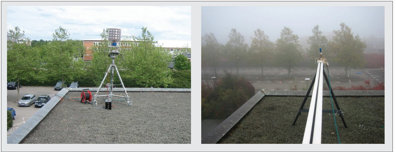
Figure 5. Massive MIMO antenna arrays used for the measurements.
