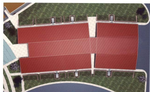
Figure 5. Aerial view of the Museum of Electrical Technology
