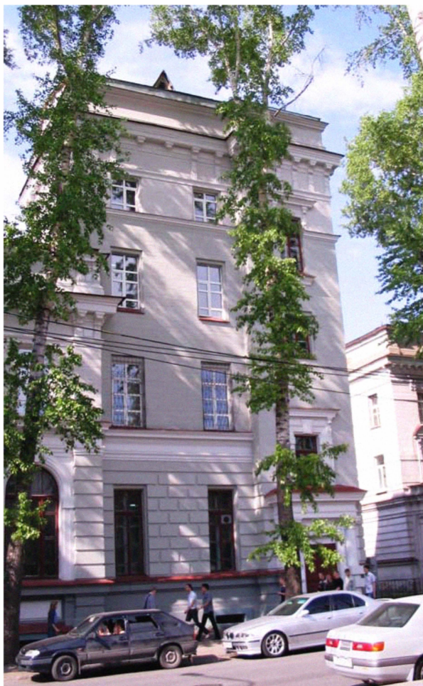
Figure 1. The physics building of the Tomsk Polytechnic Institute where on the top floor the first TV transmitter was made (so it looks nowadays).
