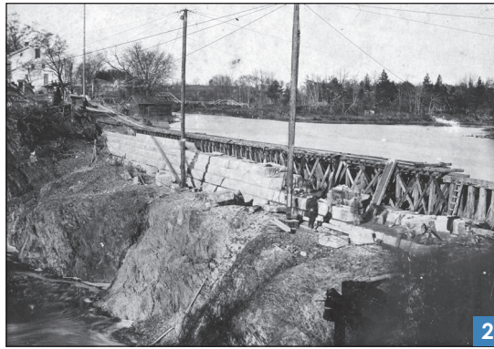
Building the new dam below the remains of the 1827 timber dam.
