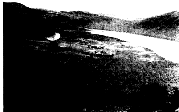
Figure 10. The completed antenna near Goldstone Dry Lake.
