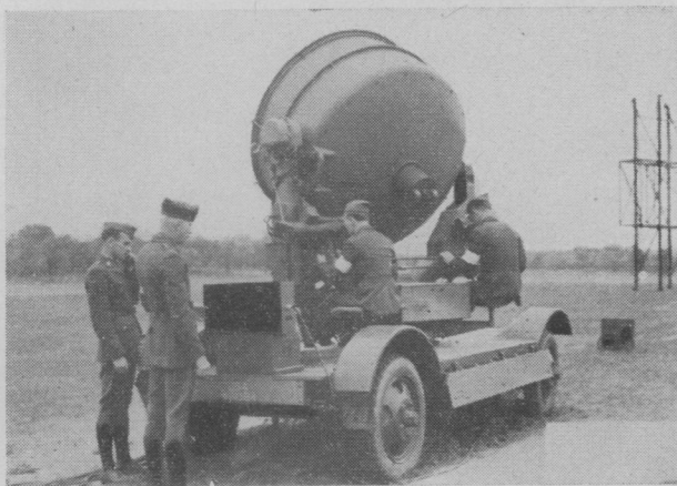
Fig. 11—Detailed view of radar and thermal-control unit. May, 1937, tests.
